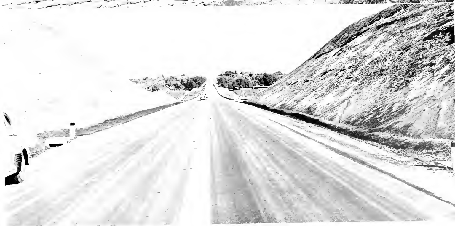
Top and bottom pictures show sections of revised alignment on State Highway between Fresno and Yosemite Valley. Center—Reinforced concrete bridge over San Joaquin overflow connected with Lanes Bridge by 255-foot fill. The bridge is 200 feet long
